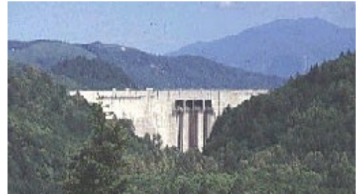
Mossyrock Dam. Photo: Tacoma Power.
