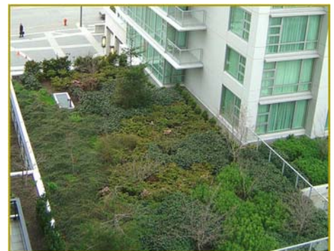
Green roof, Courtesy PNWRA
